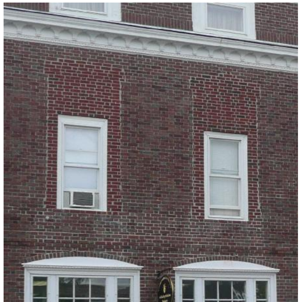
Enlarging or downsizing window openings is not appropriate. Replacement windows must be designed to fit existing window openings.
