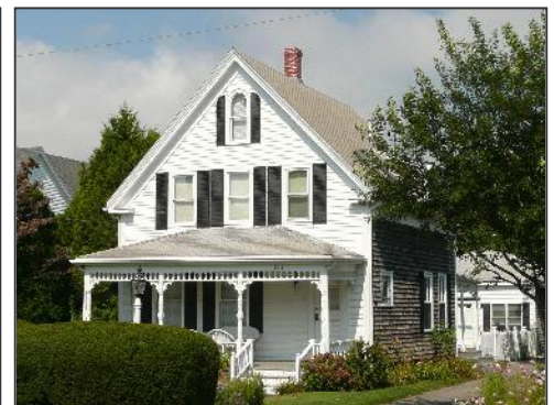
A Queen Anne style home, built 1876, sided with cedar clapboards and shakes.
